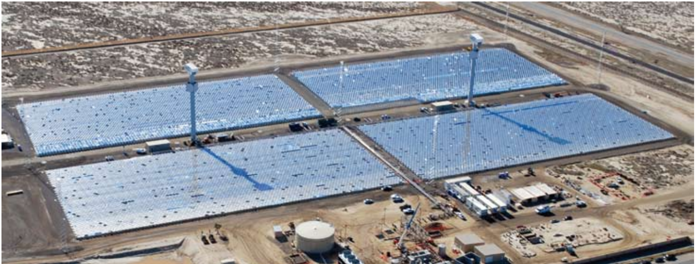
Aerial view of the eSolar demonstration solar plant in California
