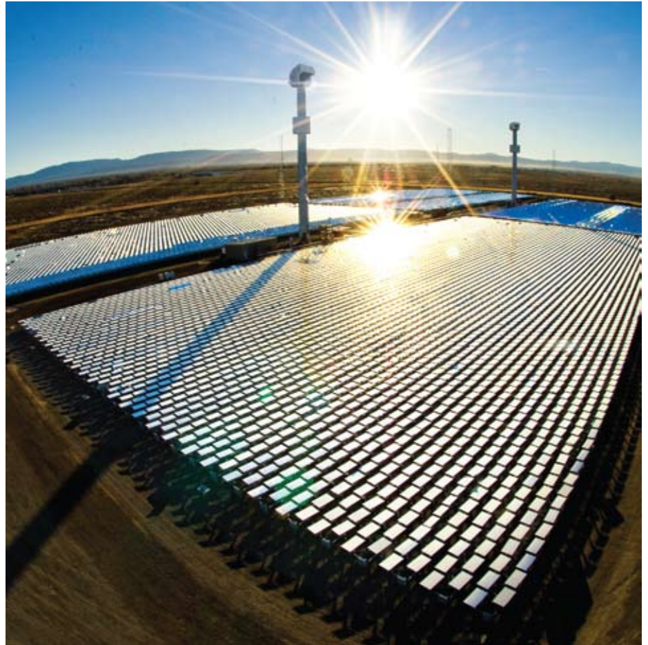
The eSolar demonstration solar plant in California showing all 24,360 heliostats, the two central thermal receivers with targets, and the towers mounted with the Prosilica cameras.
